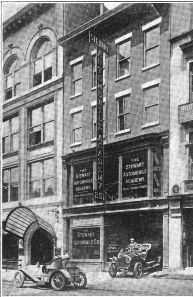
Exterior of Stewart Garage, New York City
